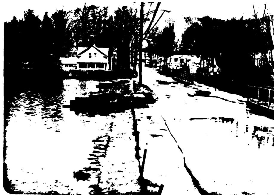
PHOTO 1 - General view of crest of dam, showing the two spillways, boardwalks and dike at left end of dam.
