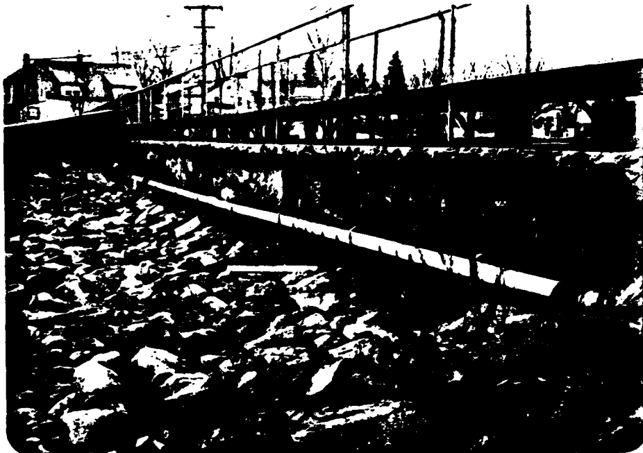
PHOTO 5 - Downstream face of right spillway. Note gas pipe along masonry wall, and potential for obstruction due to boardwalk and fence.
