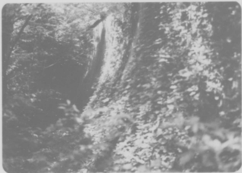
PHOTO #13: Downstream face of the concrete dike.
