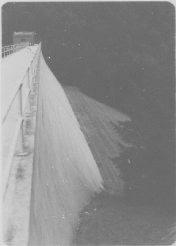
PHOTO #2: View along the face of the dam, looking east.
