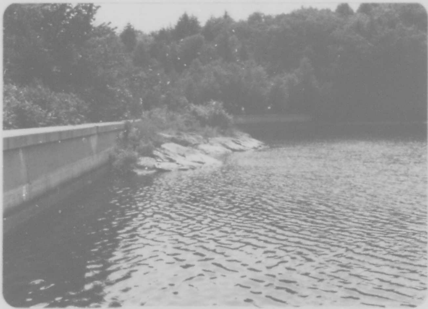
PHOTO #11: View looking south along the concrete dike.
