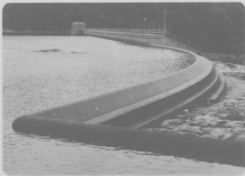
PHOTO #6: View of the spillway and dam, looking east from west abutment.
