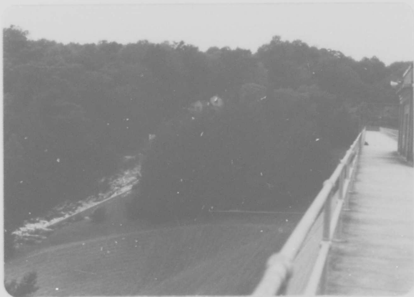
PHOTO #3: Looking west along the crest of the dam.
