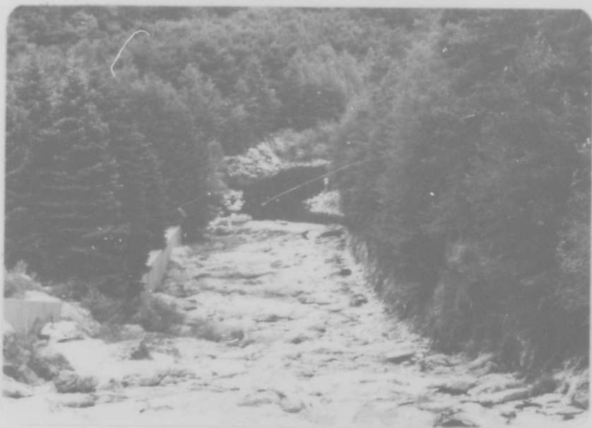
PHOTO #7: The spillway discharge channel, looking down at the natural river in the background.
