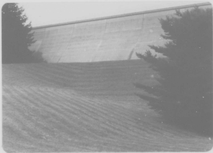
PHOTO #1: View of the western, downstream face of the dam.
