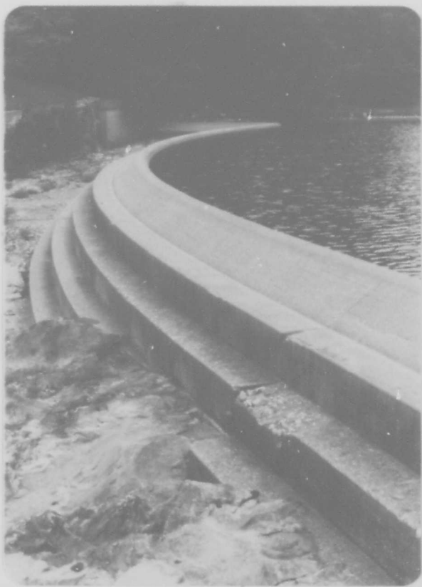
PHOTO #5: View of the spillway, looking west.
