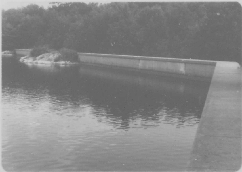
PHOTO #12: View looking north along the concrete dike.
