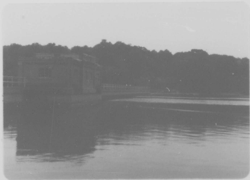
PHOTO #4: Upstream face of the dam and upper gate house.
