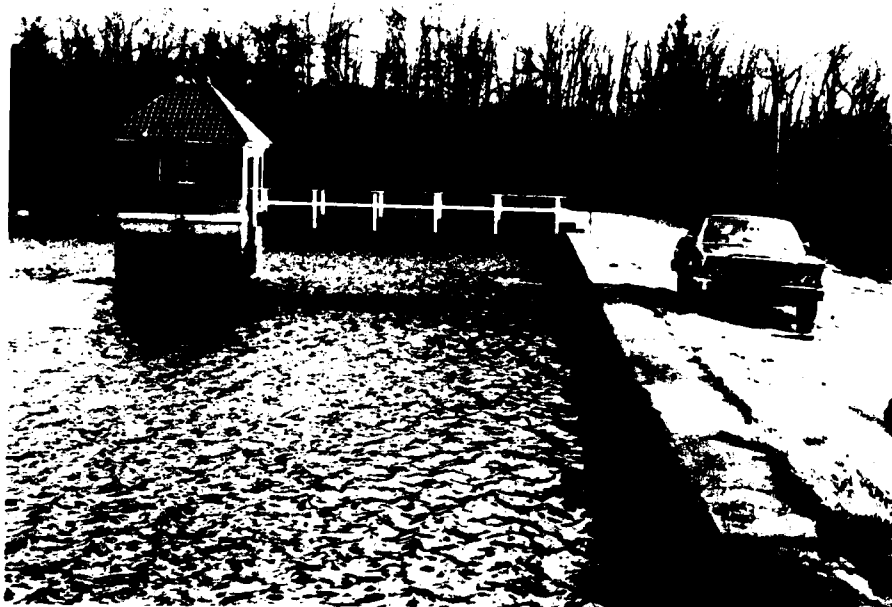
C-2 DAM CREST AND GATE HOUSE - LOOKING EAST
