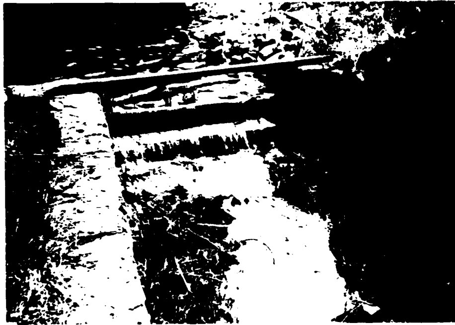
Photo 7 - Upper spillway weir with stop-planks and spillway channel (May 1979)
