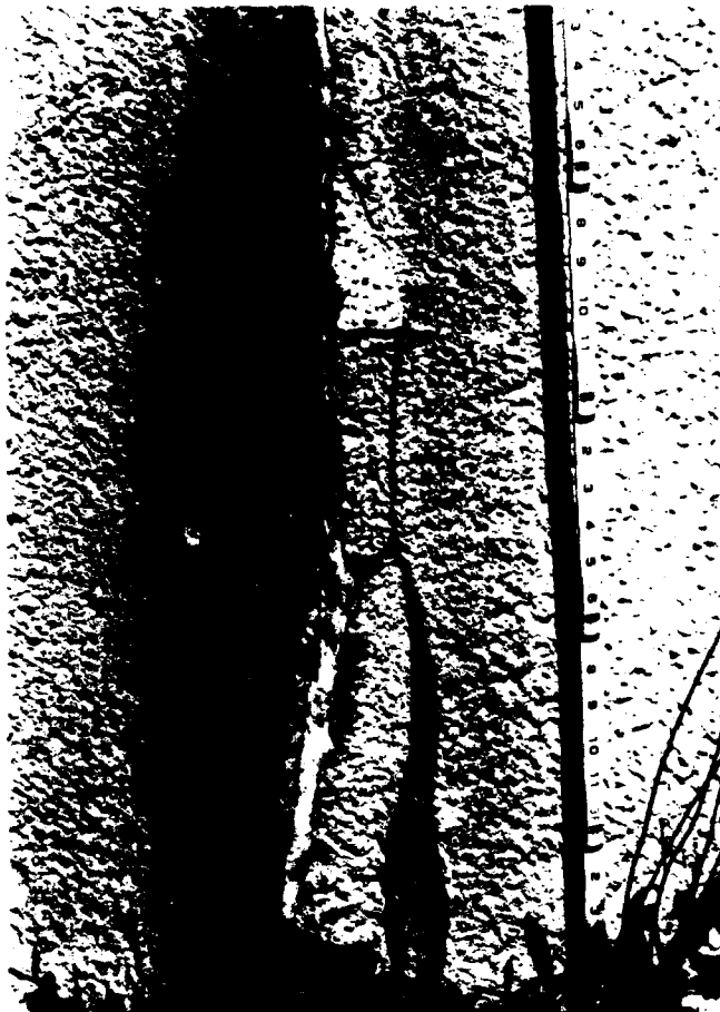
PHOTO #11: Typical Spalling at Joint, Downstream Face.
