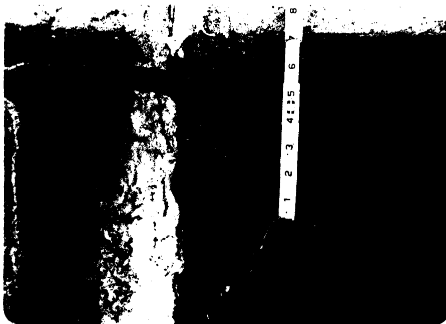
PHOTO #10: Typical Spalling at a Construction Joint on the Upstream Face of the Dam.
