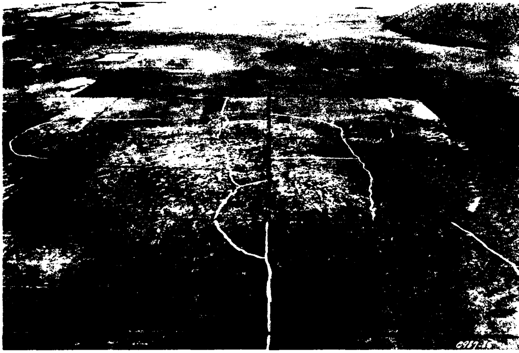
Photo 33. Item 10 after 2500 passes and 500 turning movements
