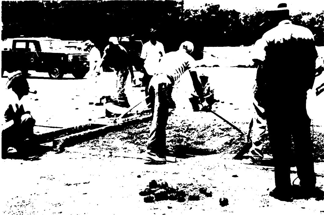
Photo 5. Placing fibrous concrete in item 3
