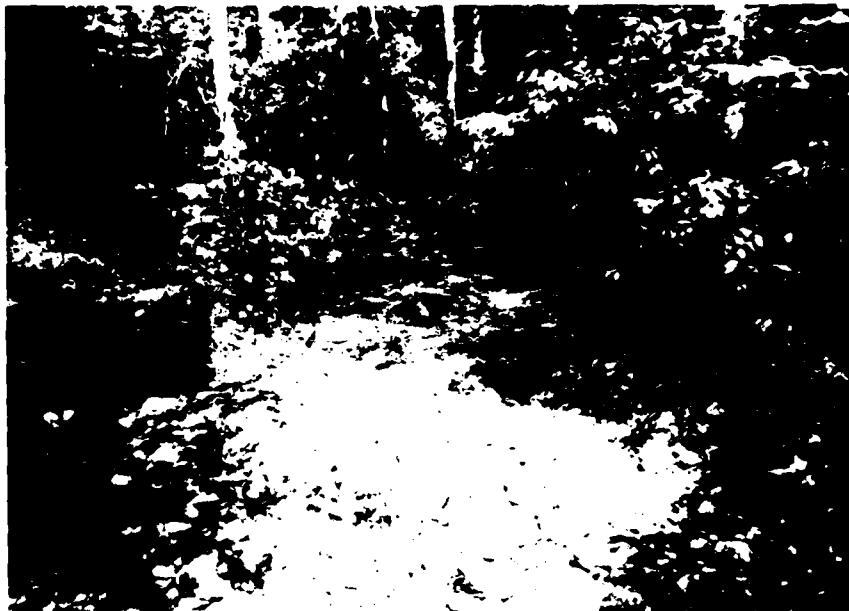
Photo 11 - Spillway discharge channel from upstream. Note boulders, ruts and trees on channel floor. (Aug 79)
