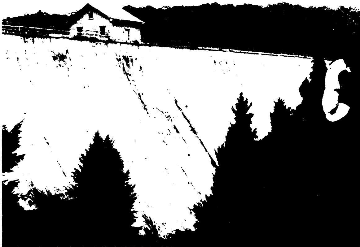
EASTON RESERVOIR DAM
