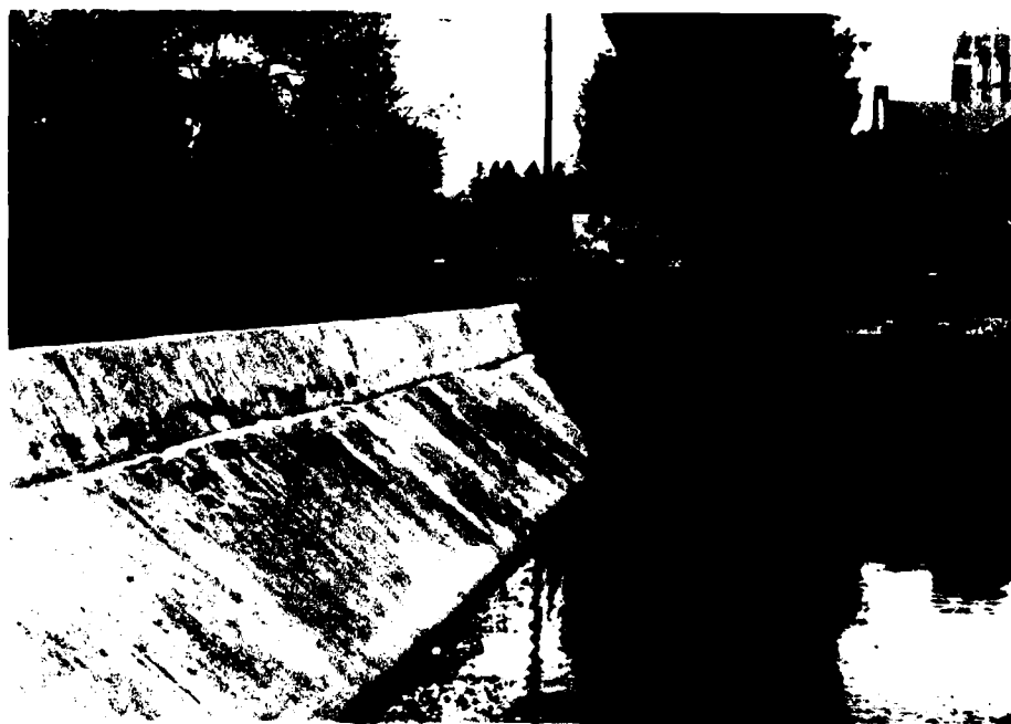
PHOTO #4: Upstream face of dam looking towards right abutment. Note 3-foot parapet wall on top of concrete face and earth embankment at right side of dam.
