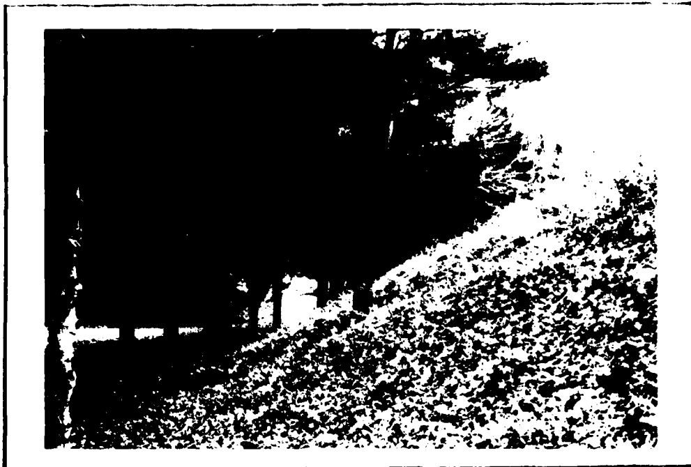
5. DOWNSTREAM FACE OF THE DAM NEAR THE LEFT ABUTMENT SHOWING TREES GROWING ON THE EMBANKMENT. (11/13/79)
