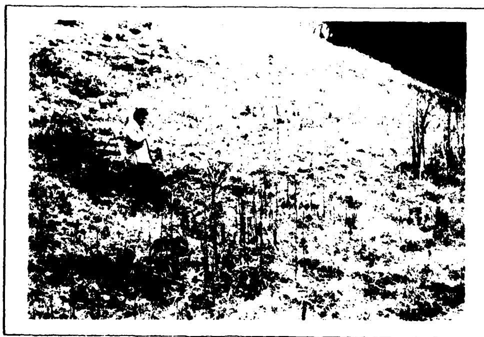
2. DOWNSTREAM FACE OF THE DAM SHOWING VEGETATIVE COVER AND A DEPRESSION IN THE EARTH EMBANKMENT. (11/13/79)
