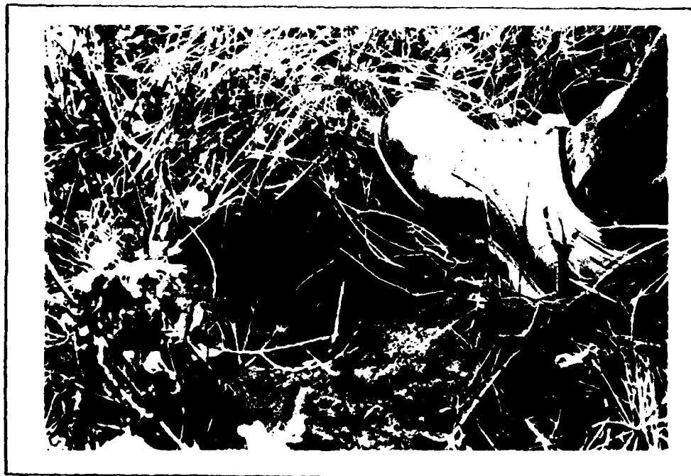
4. TYPICAL RODENT HOLE IN THE DOWNSTREAM FACE OF THE DAM. (11/13/79)
