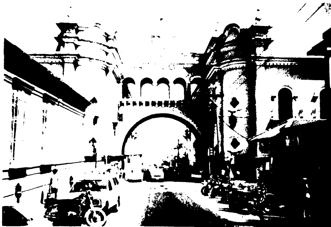
Post Office, Guatemala City Courtesy James D. Rudolph
