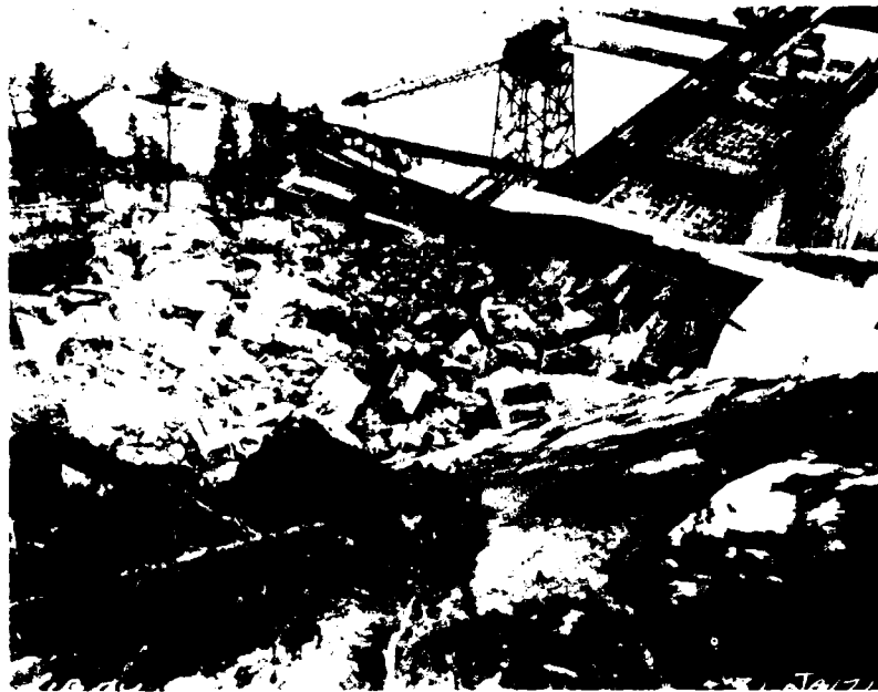
3.11a View down slide along surface of the Dirty Shame +122 Bedding Fault to rubble pile. Refrigeration plant on right, aggregate cooling facility right center, uncompleted dam upper right.
