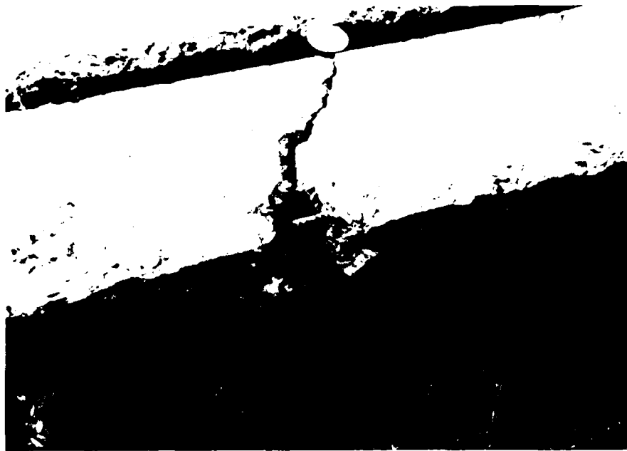
Figure 41. Close-up of beam 149. Note severed rebar
