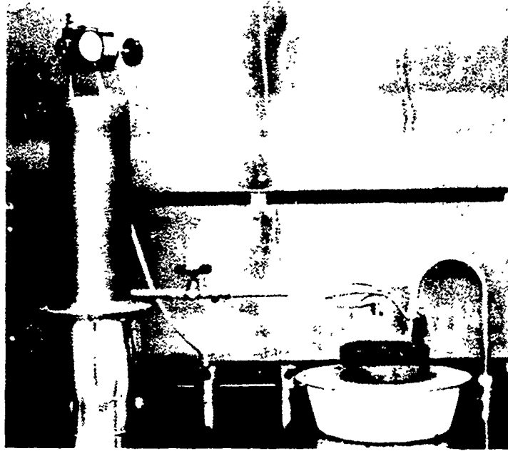
Figure 4. Fuel-Drip Test Device.
