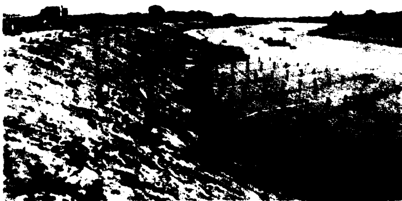
BELOW: Wire fence dike field. Note that the top of each fence post is guyed to the bottom of the fence post immediately upstream and that each fence line is tied into the bank.
