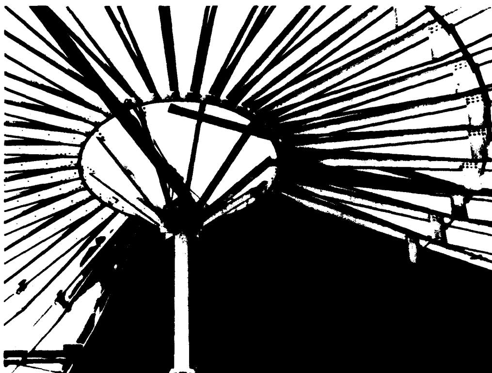
Members of the 811th Engineer Aviation Battalion lay the cover sections of a petroleum storage tank at a Korean base.
