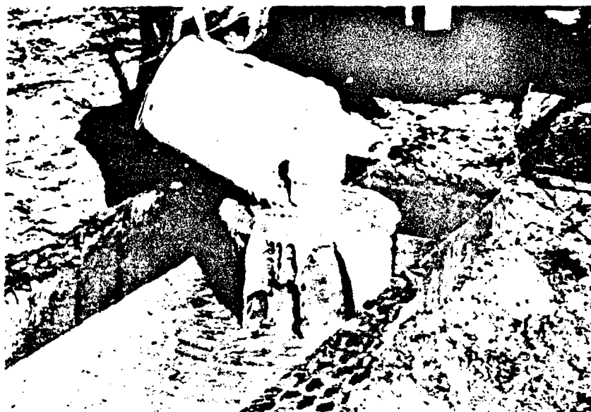
PHOTO E Pouring bentonite pellets into hole for seal above gravel pack at Main Base.
