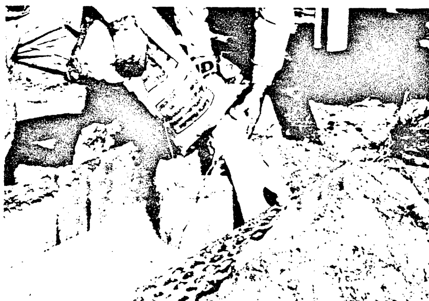
PHOTO D Pouring sand into hole for gravel pack around the screen.
