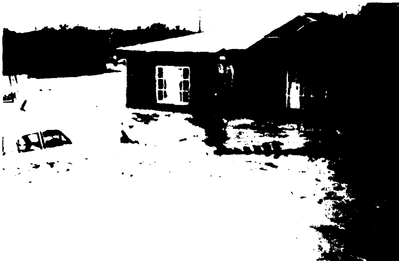
Photo A-5 (cont.). Flooding south of river in 1970
