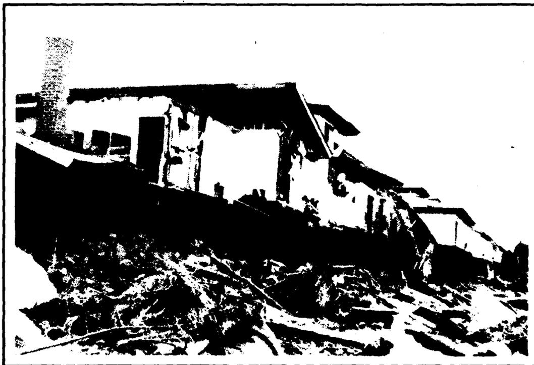
Photo 11: Floodwaters undermined houses next to Santiago Creek during the 1969 Flood.
