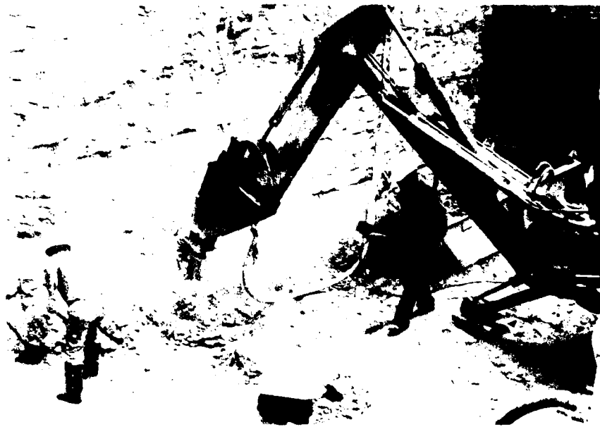
Figure 6 Rock excavation using jack-hammer mounted on back hoe
