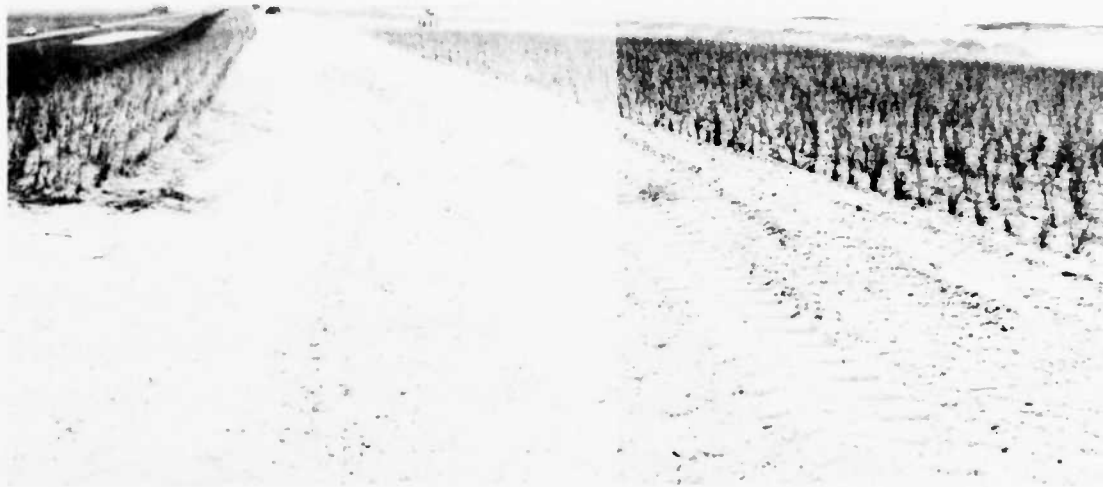
Fig. 12. The dike with the road to the left north of Torsminde photographed towards south in April 1983. The dike is under re-construction. Heaps of building materials are seen on the beach. The dark spots to the far right are artificial boulder reefs. The dike is planted with Marram Grass to prevent aeolean sand transport.
