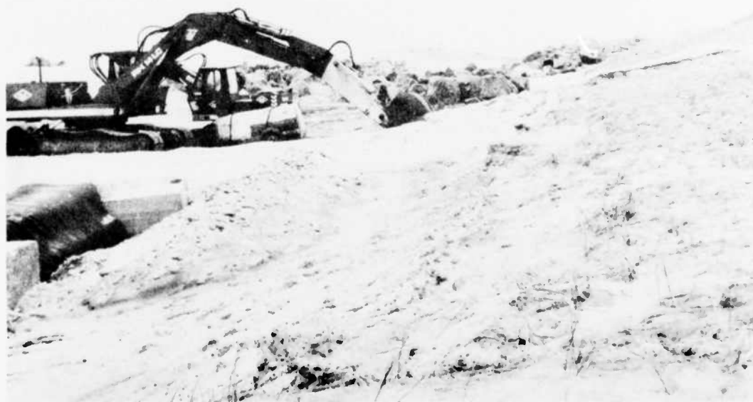
Fig. 13. Constructional works on the northern part of the barrier seen from the south in April 1983. The dike has newly been re-established and planted with Marram Grass, but the foot of the dike has recently been strongly eroded. A wall, supporting the foot of the dike, is under construction. Such measures have to be carried out along a shoreline of 18 km. See also Fig. 12. In the far background the groyne Q can be seen.
