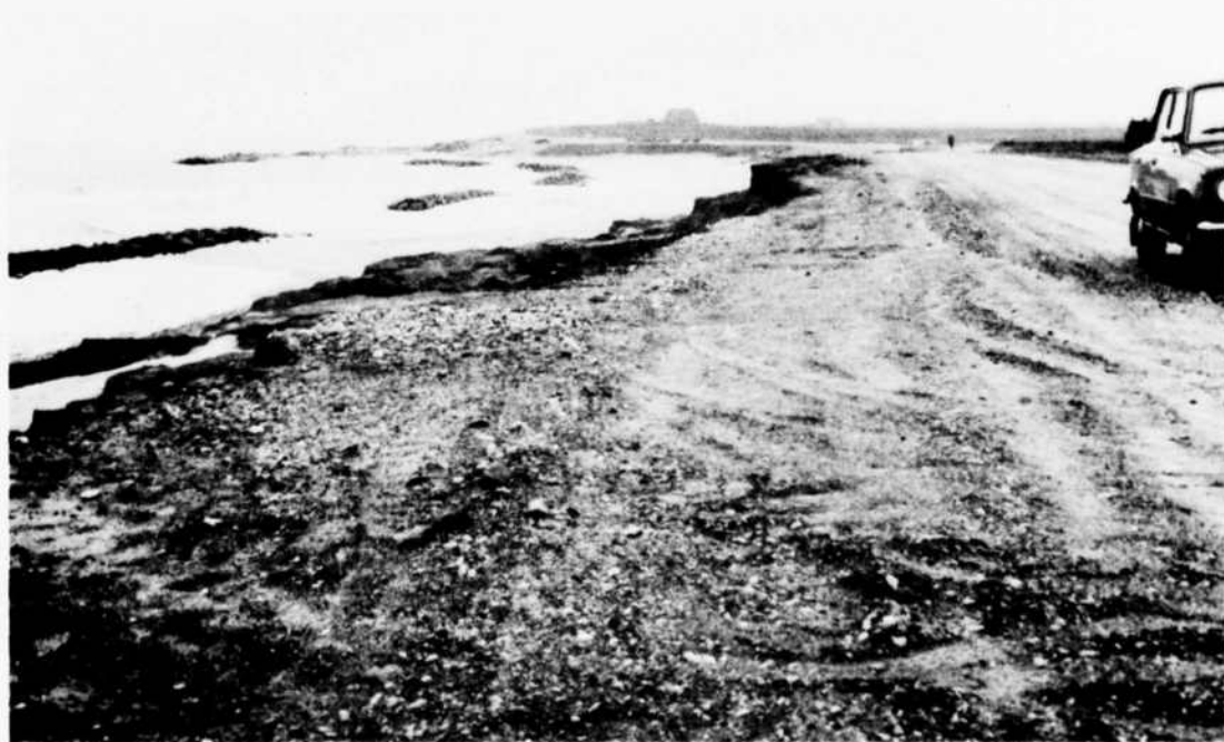
Fig. 11. Groyne Q in the background opposite the houses seen from the south in April 1983. The small embayment, eroded on the lee side of the groyne, is clearly seen. On the beach heaps of basalt boulders have been placed and small tombolos connecting the cliff with the artificial reefs have been created. The surface in the foreground with the eroded side, facing west, is an artificial coastal cliff built in attempt to protect farming land and houses opposite point 3, Fig. 2.
