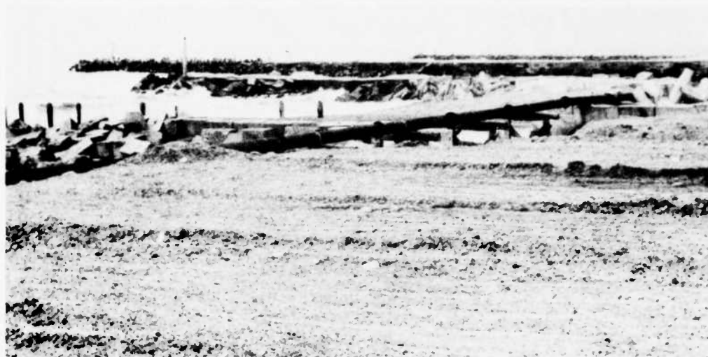
Fig. 6. The outlet to the North Sea from Nisum Fjord seen from the south in April 1983. The short jetties flanking the outlet are seen in the central part of the photograph. In the far background the groyne north of the outlet (5, Fig. 2) can be seen. The surface in the foreground has been built up artificially. The tube was placed in connection with experimental works on nourishing the beach south of the outlet with sand, dredged in the fishing port.
