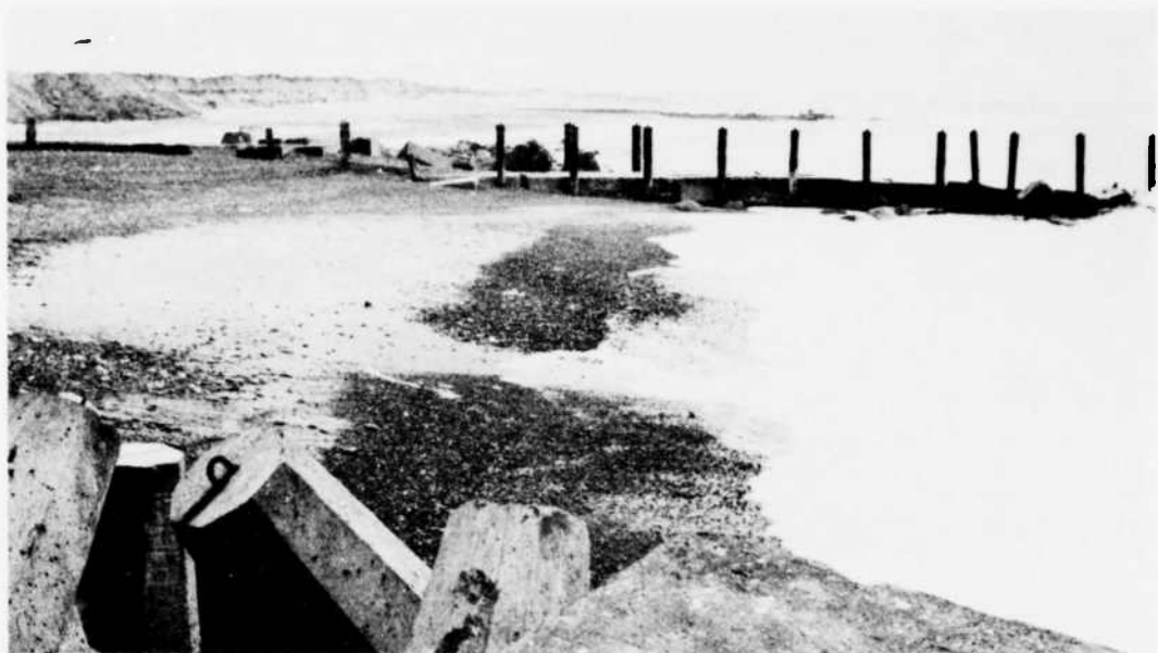
Fig. 8. The coast south of the outlet at Torsminde seen from the southern jetty in April 1983. The coastal cliff has been supplied with gravel, but in the background the eroded cliff can still be seen. The groynes (Fig. 2, 8 and 9) are constructed 1939-45 in an attempt to prevent erosion south of the outlet. It is clearly seen that the groynes did not work. The beach- and cliff nourishment is very expensive, but the harbour basin is situated just 150 m east of the cliff (Fig. 5). The material for beach nourishment here has been excavated north of the northern jetty, thus reducing the transport of sediment ending up in the outlet.
