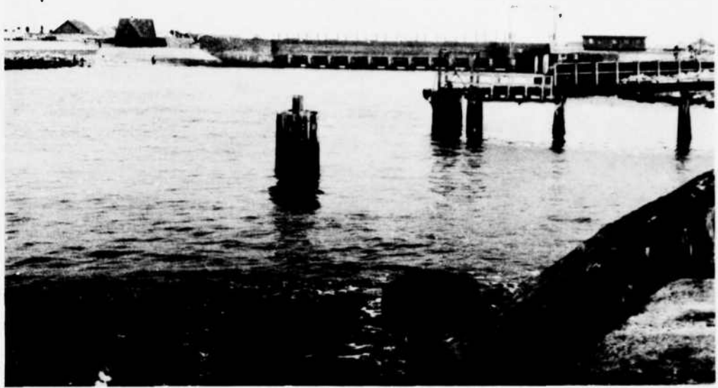
Fig. 4. The sluice at Torsminde with all valves open, seen from the southern jetty in 1983. The sluice was constructed in 1868-70 and controlled the outlet until 1889. Then it remained abandoned and isolated until 1931 in which year the sluice was extended with two sluice valves and a shiplock and re-opened. The gantry crane to the right lifts the lock gate, on the photograph hanging halfway in the water. The entrance to the present fishing port is to the far right.
