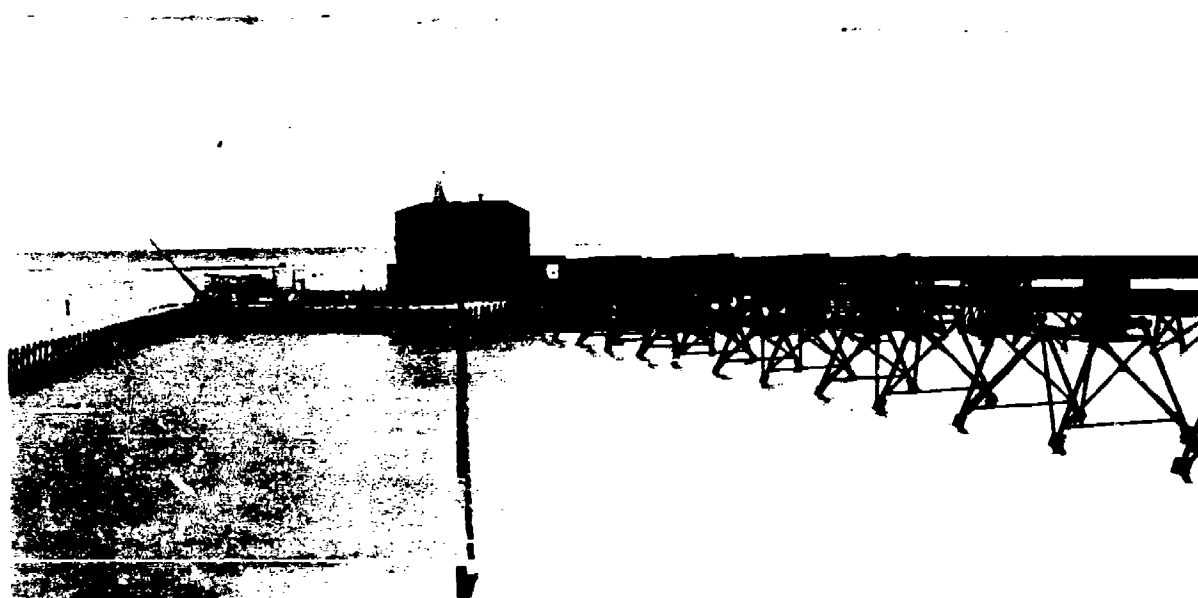
Figure 2. Surface detonation cab, showing pipe array for diagnostic experiments, REDWING.
