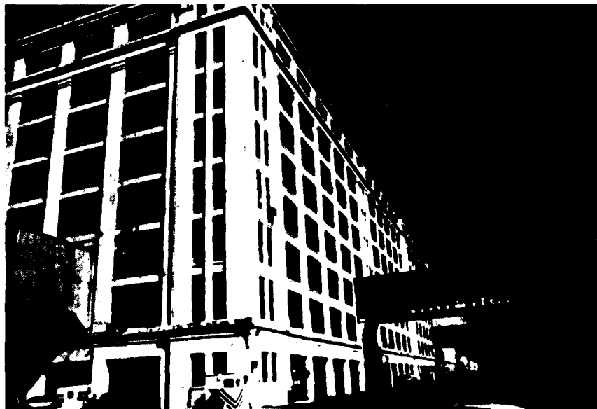
Plate 55. Facility 2, 666 Summer St., Boston, Mass. The marine supply terminal at 666 Summer Street.
