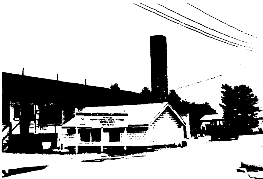
Plate 2. Facility 1, Bldg. P-211, Fort Devens, Mass. The Steam Heating Plant. Built in 1917 at Fort Devens, Massachusetts. It has been converted to oil.
