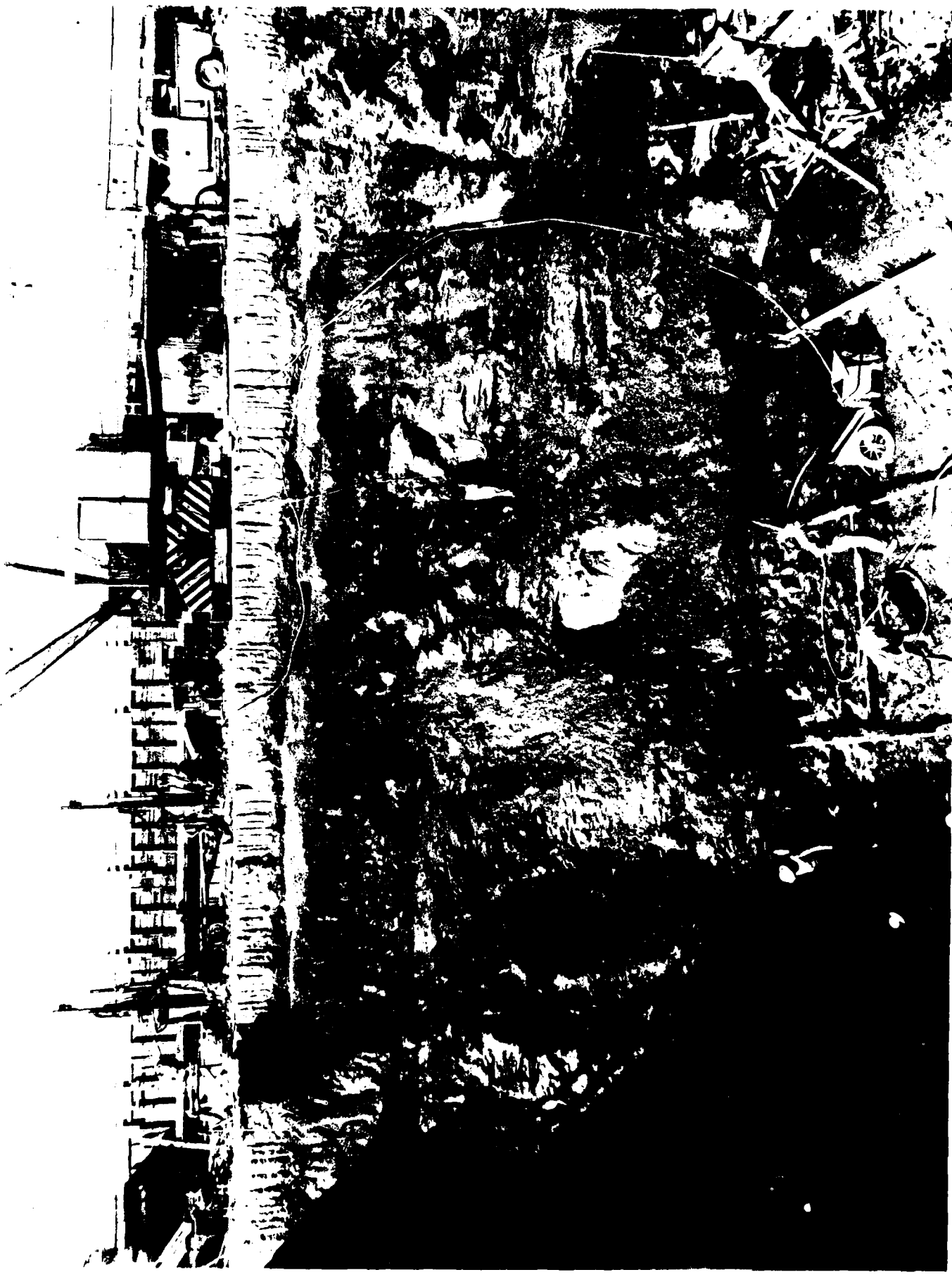
Photo No. 31 Foundation, Powerhouse No. 2, Area N. Showing 3A Fault (Pointed to by Man on face). Fault dips NE 52^{\circ} stake NW to SE.
