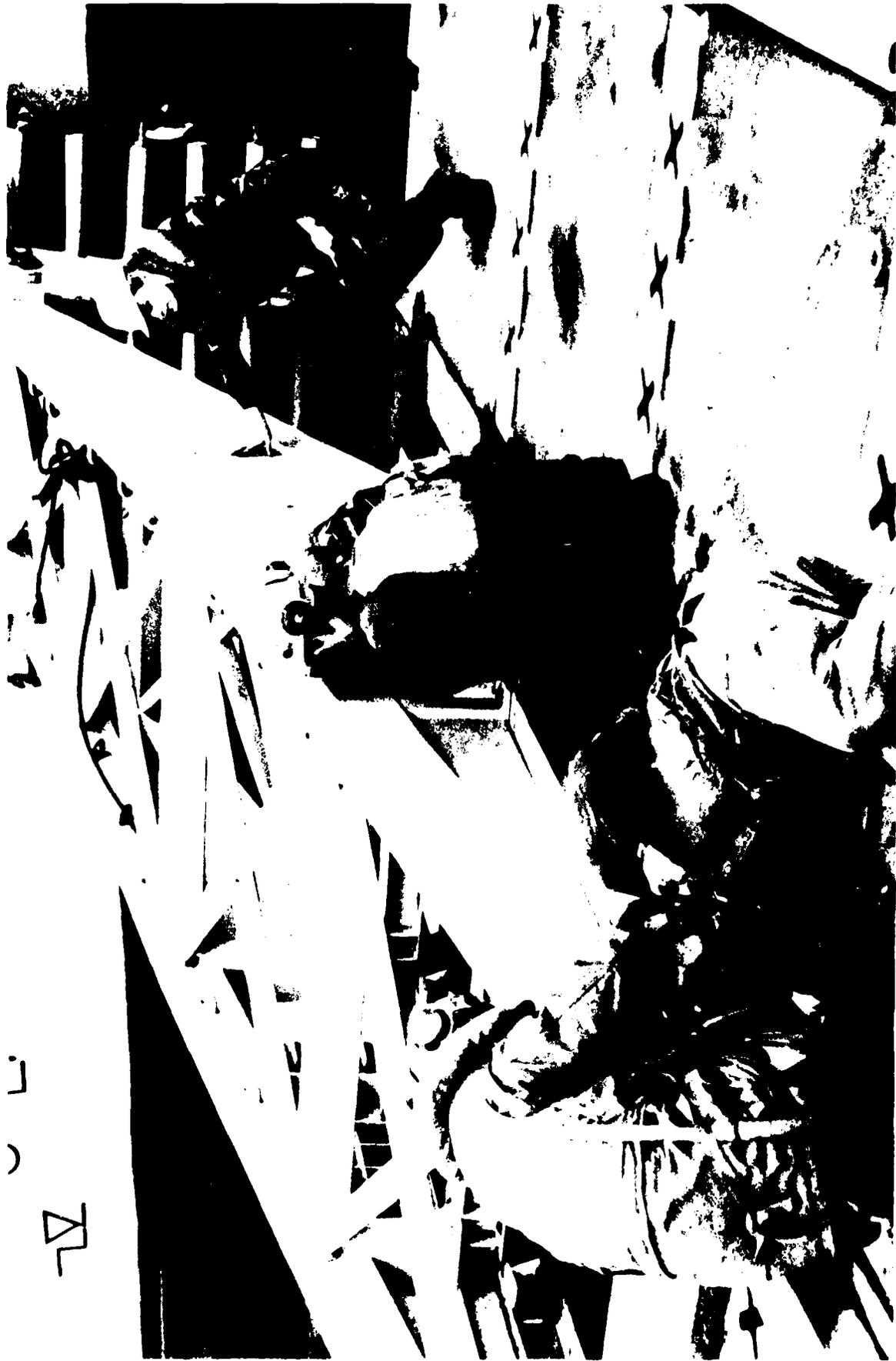
Figure 48 - Fender Bolts Being Tightened to Reduce Movement
