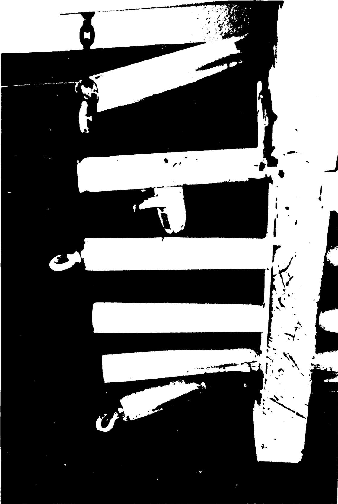
Figure 41 - Result of Fender Contact with Ship (View 1)
