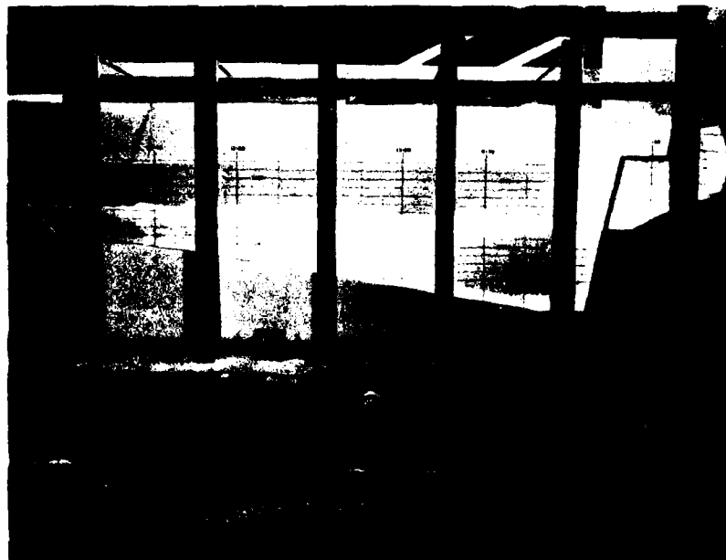
Photograph 12. Discharge per bay 5,700 cfs; river discharge 28,500 cfs; tailwater elevation 2081.00
