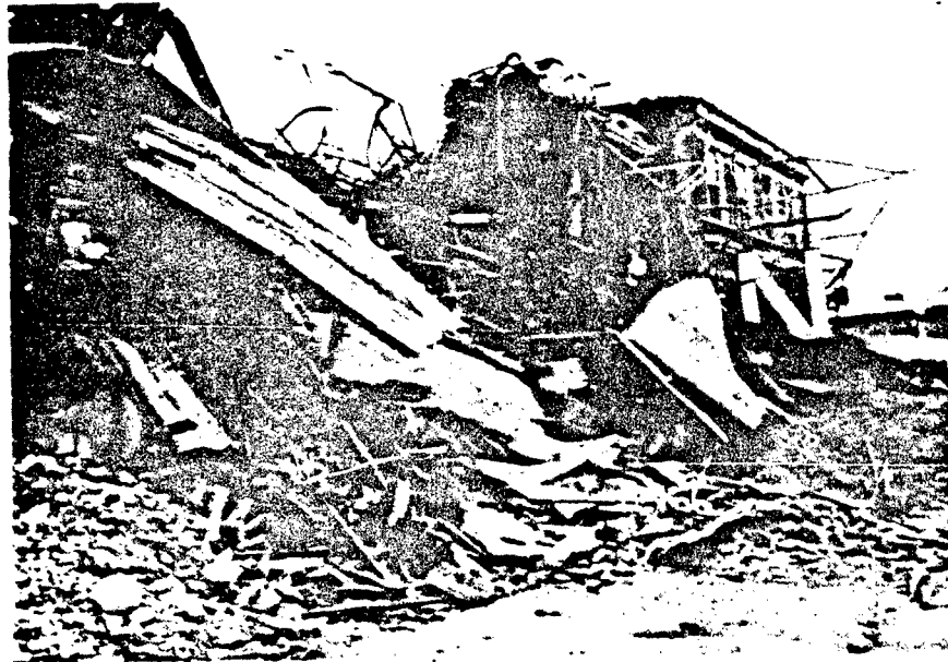
Fig. F-7. Debris Pile From the Newhouse Hotel in Salt Lake City, Utah.
