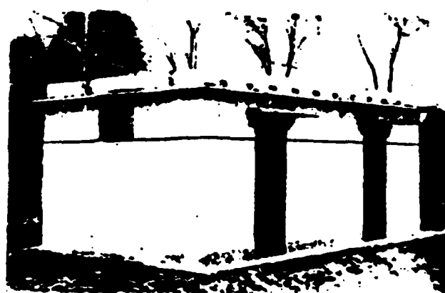
Photo 9. "System 768" earthquake station
