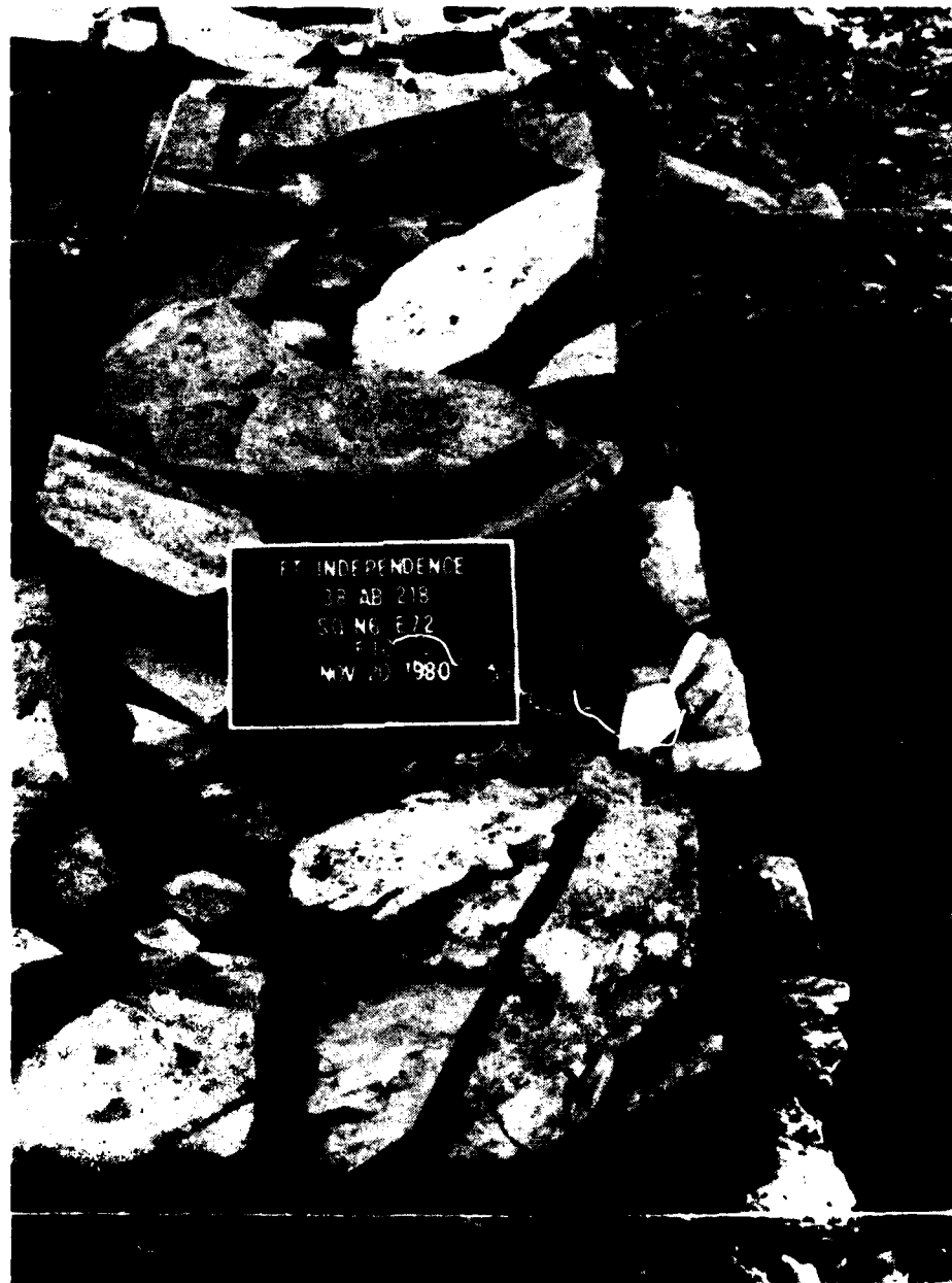
Figure 13. Example of stone masonry, rear of Feature 10, looking south.
