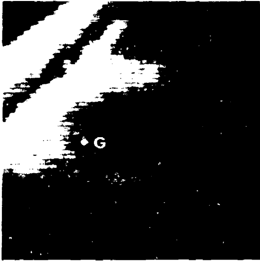
Figure 12. Thermogram of a bright area along the penthouse flashing.
