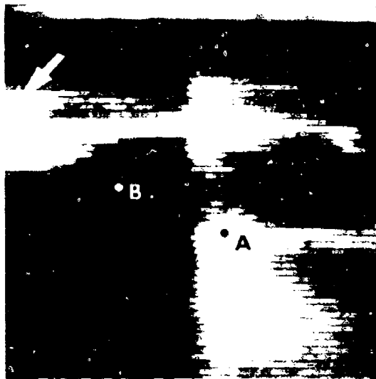
Figure 8. Thermogram of a 2-ft-wide thermal anomaly extending from the roof edge to the monitor. The arrow points to a roof drain.
