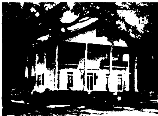
Figure 30. Cox house, Stockton, Baldwin County, 1870s.
