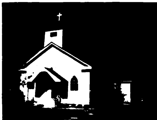
Figure 50. First Methodist Church, St. Stephens, Washington County, 1857.
