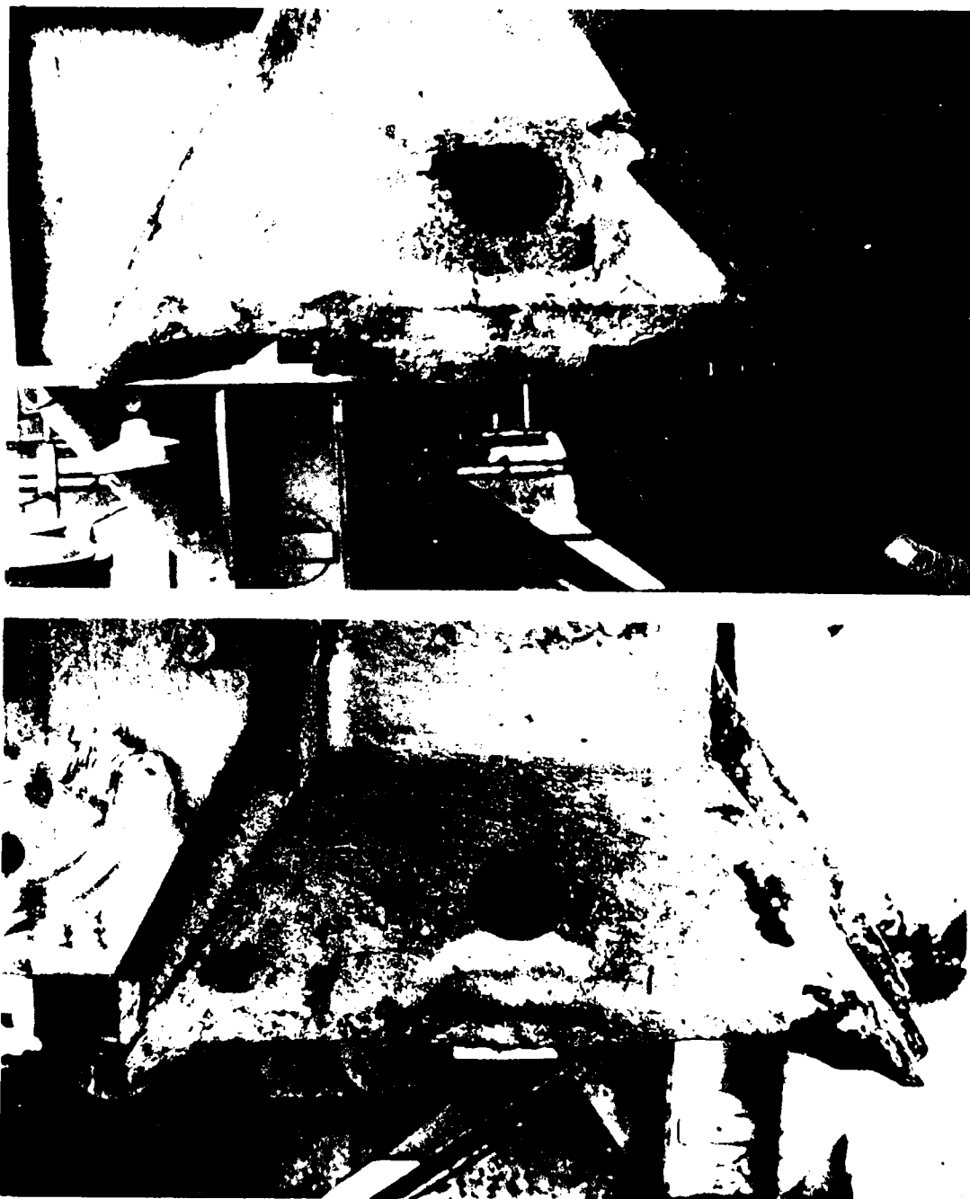
F.11a and F.11b. GATHERING CONES BEFORE AND AFTER MODIFICATION. Photo at the top shows the cone before the lip was cut off and the photo at the bottom shows the results after a cut was made. The decision to cut them and the subsequent modifications to each of the four cones delayed loading for approximately 24 hours.
