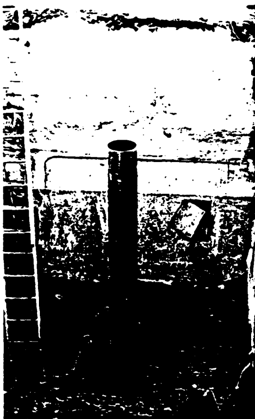
PHOTO A Extension of well casing
