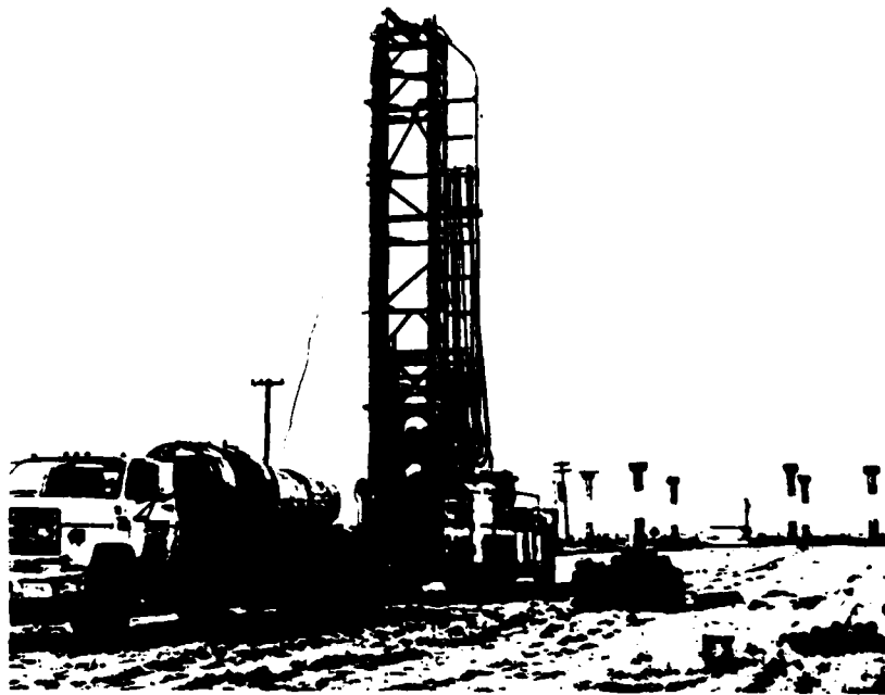
PHOTO B Rotary-wash drill rig and water tank at MW38D
