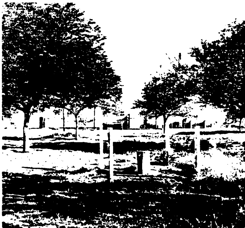
PHOTO B Monitoring Well 27S,D with locked iron casing and wooden posts
