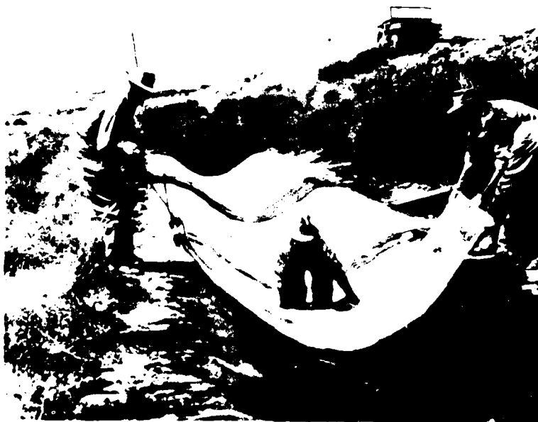
Figure 46. Lining ditch with prefabricated asphalt panels.
