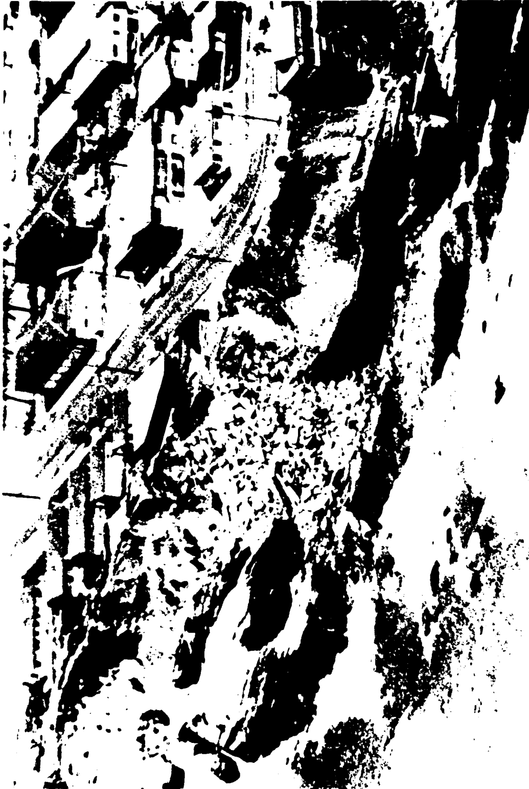
Figure 2. Random miscellaneous dumped soil, rock and rubble fill used as shore protection, Sunset Cliffs, San Diego, California (photo courtesy of the City of San Diego).
