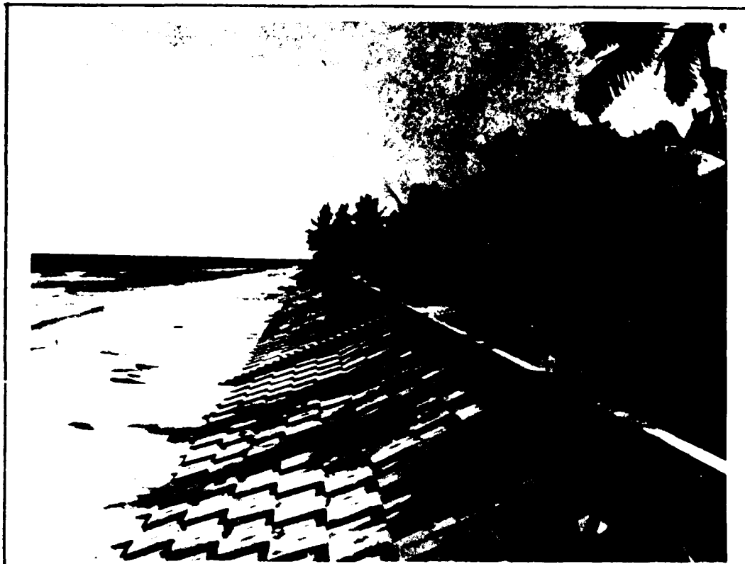
Jupiter Island, Florida (1965) Courtesy of Carthage Mills Inc. Erosion Control Division
