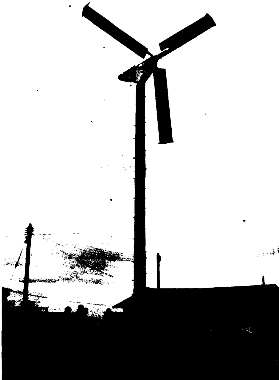
Figure 4. WECS wind turbine generator at MCAS, Kaneohe Bay, Hawaii.
