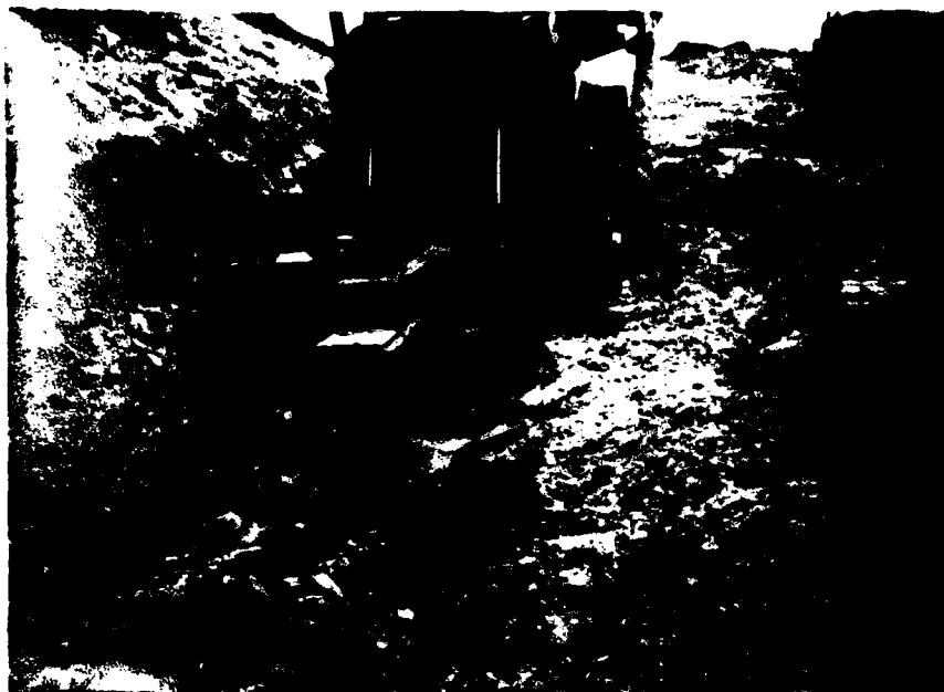
Ripping neat and sanded grout. 8 ft \pm above SS - LS contact
