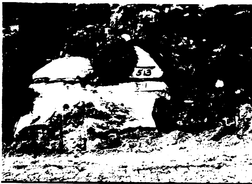
US wall Sta. 1+30 to 1+50. Extensive solutioning with clay filling. Abundant grout at lower SS contact. Dike embankment in foreground.
