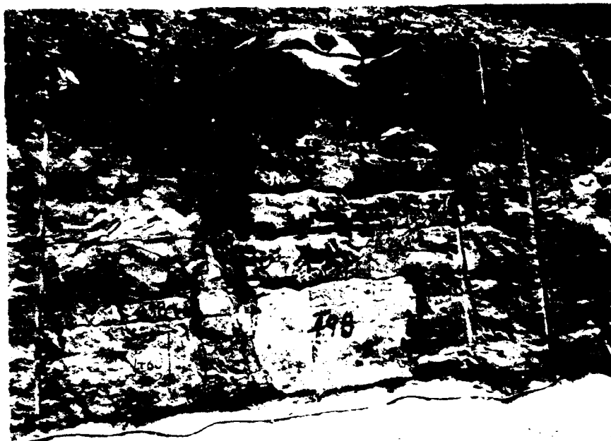
DS wall in LS Sta. 1+50 to 1+80. Note solutioning activity. Also note greenish shale at bottom of photo.
