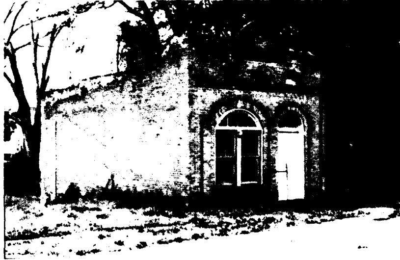
Figure 15: The Lowndesville, South Carolina, Bank (Photo: THG)
