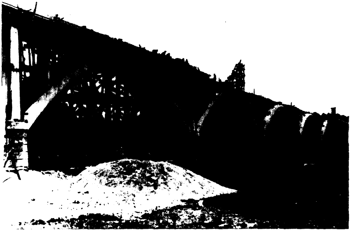
Figure 20: The Georgia-South Carolina Memorial Bridge Under Construction (Photo: Corps of Engineers)
