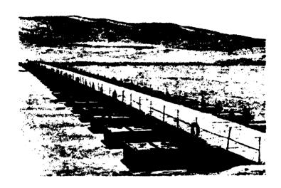
Fig. 11. Floating bridge from the pontoon train TPP.
