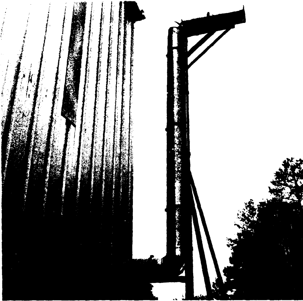
Figure 31. The Exterior Portion of the MFI Exhaust Ducting
