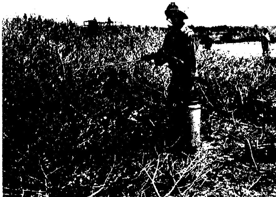
A Vietnamese soldier sprays fuel oil on underbrush to set fire as a method of vegetation removal.
