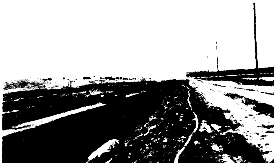
Photo No. 19 - Placement of impervious blanket in closure section, looking south. 5 Aug 1955.
