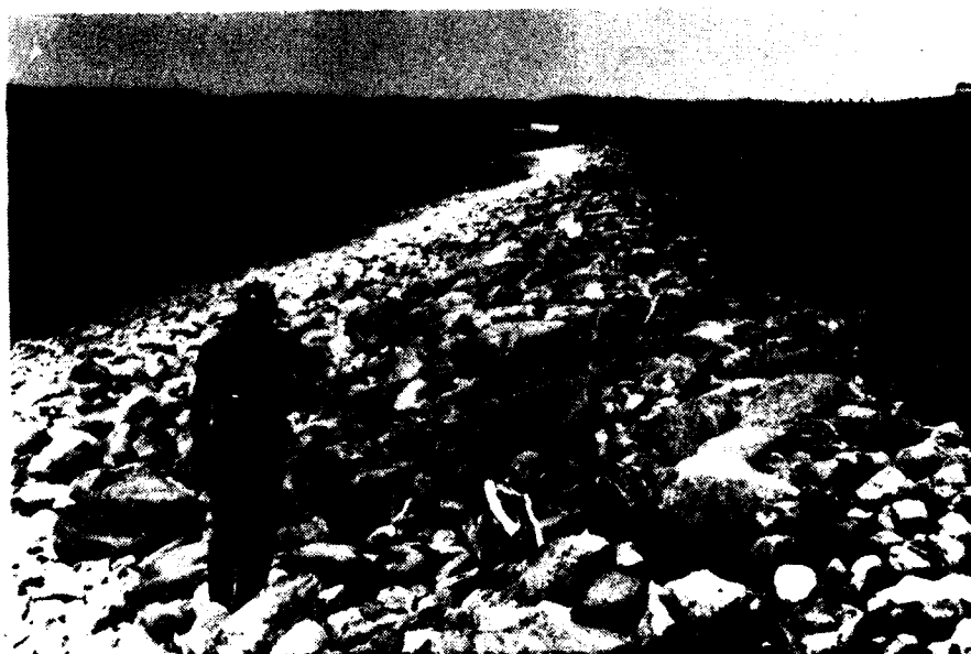
Photo No. 4 - Field boulder upstream slope protection. May 1979.
