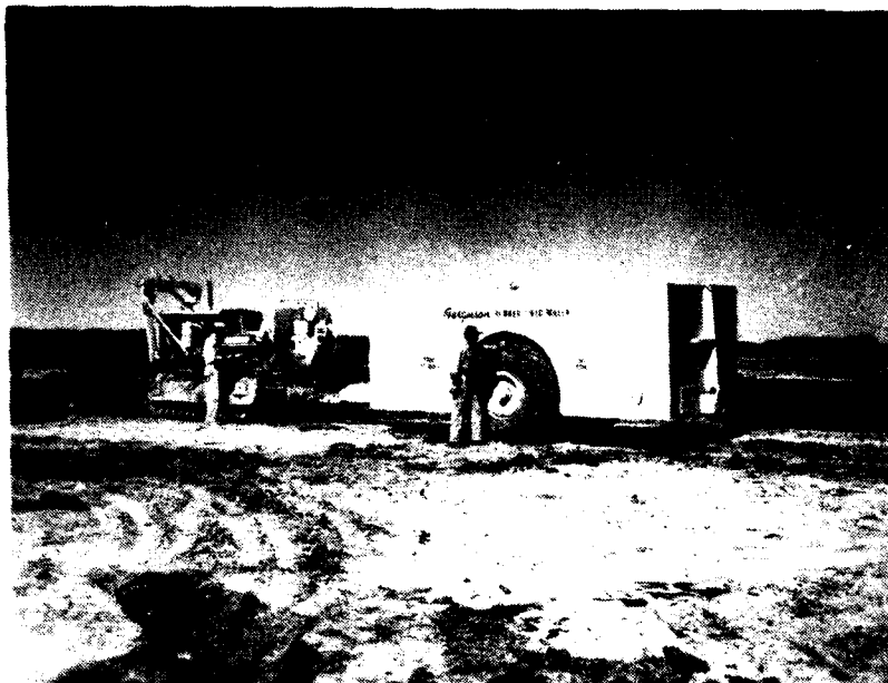
Photo No. 9 - Ferguson 50-ton rubber-tired roller used to compact embankment, Earthwork Stage I. Aug 1952.
