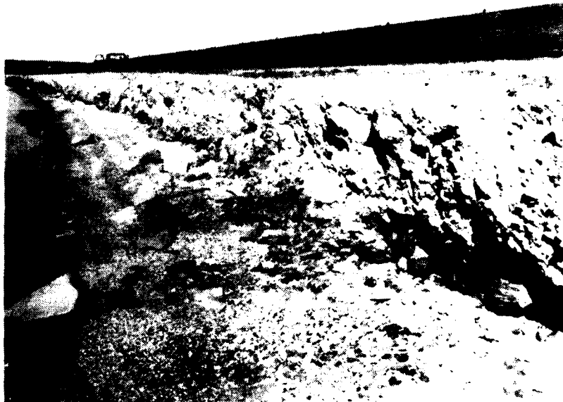
Photo No. 25 - Wave erosion scarp along embankment upstream chalk berm. Oct 1966.
