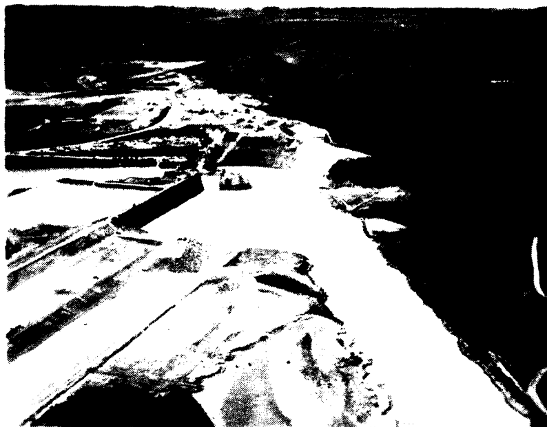
Photo No. 21 - Aerial view of south abutment area, showing powerhouse and spillway structures, the south portion of embankment, and the diversion channel. Aug 1955 (est.)
