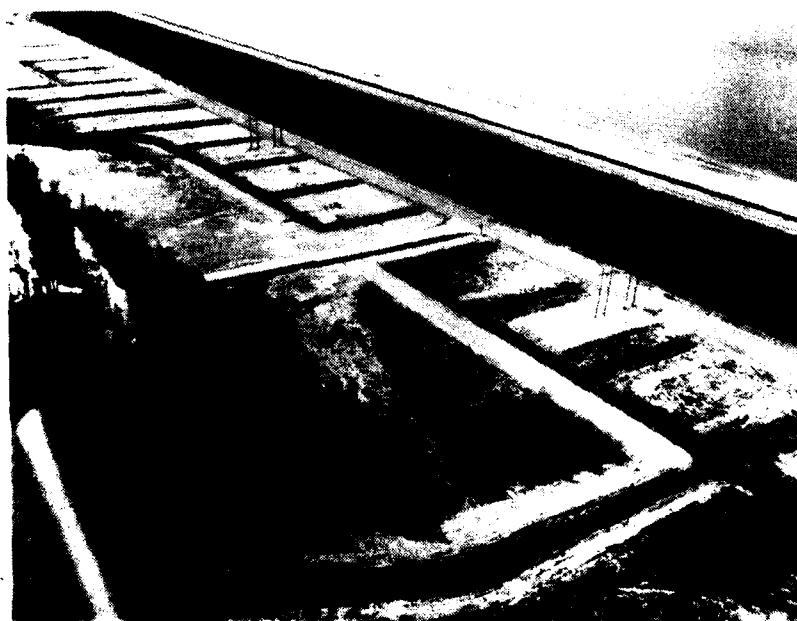
Photo No. 24 - Aerial view showing relief well discharge and collector ditches. Discharge ditch for relief well No. 19 is pictured in extreme right of photo. 8 May 1957.
