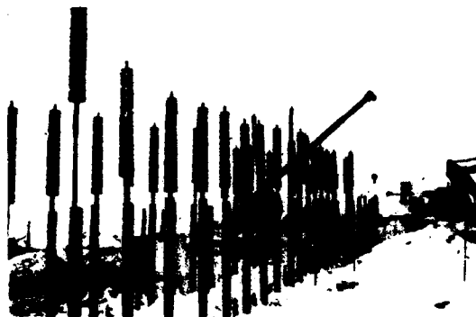
Figure 12. Completed Installation of Heat Pipes
