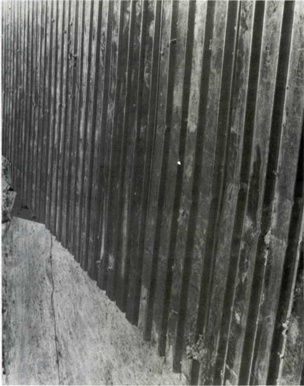
Figure 11. Damage to roof flashing
