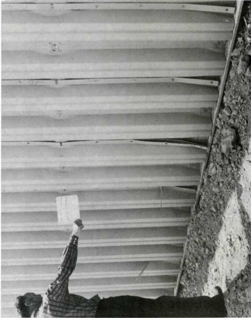
Figure 13. Pull out of panel screws
