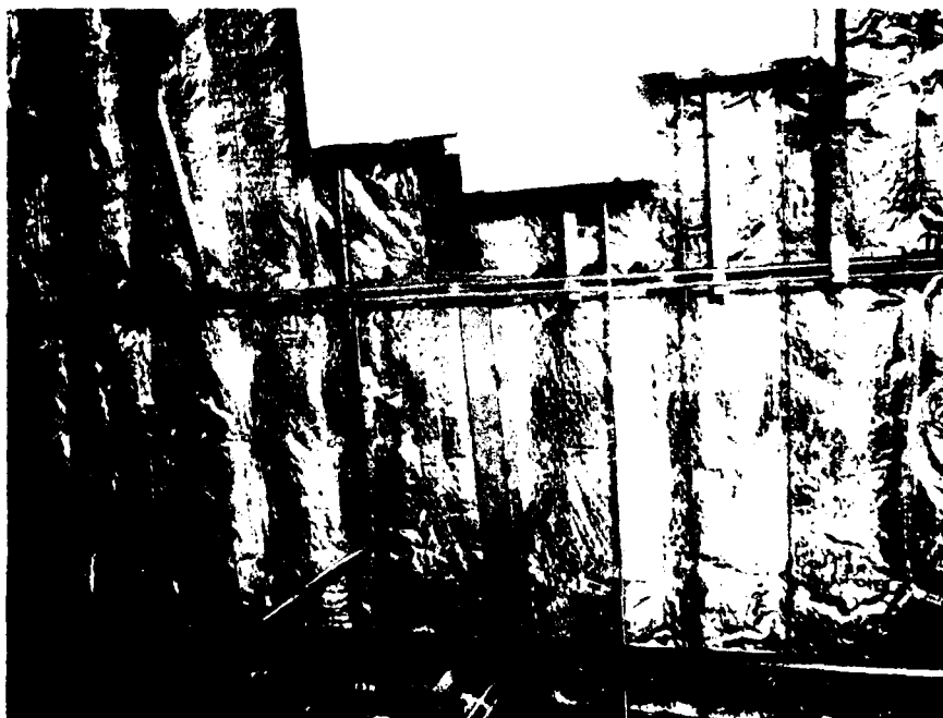
Figure 10. Insulation batts supported on chicken-wire.
