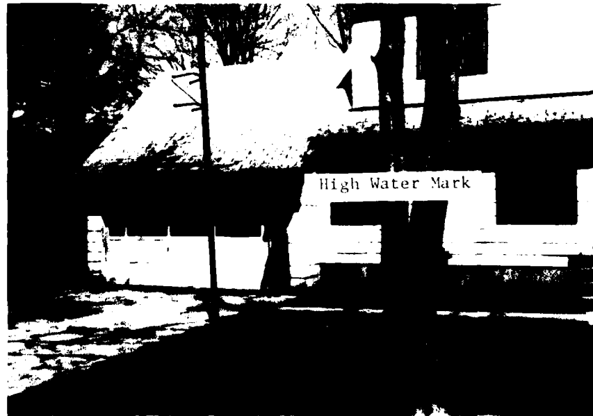
Photo 10 - Same residence as above showing high water mark. Photo taken 6 April 1978
