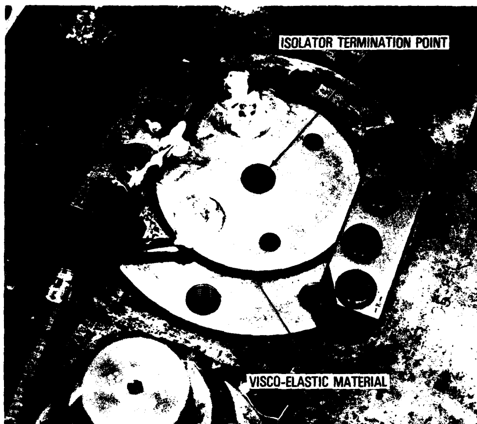
Figure 8. Vertical Terminator in the Foundation
