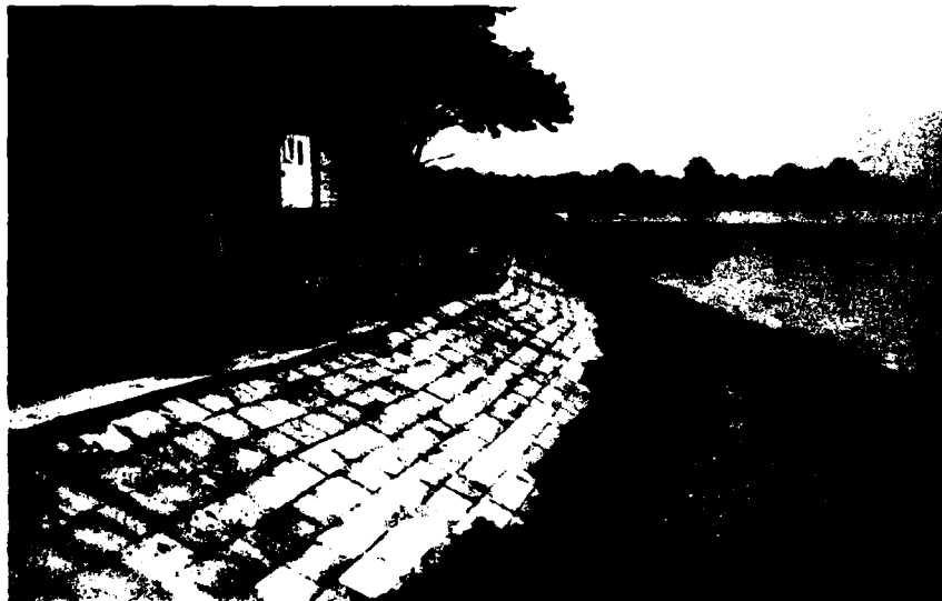
Figure 50 Shiplap Block Revetment
