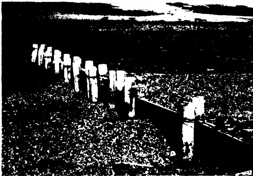
Figure 82 Timber Plank Groin
