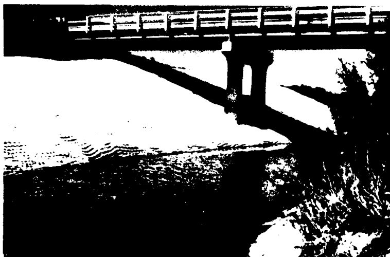
Figure 55 Grout-Filled Mattress (Fabriform) Revetment (Photo Courtesy of Construction Techniques, Inc.)
