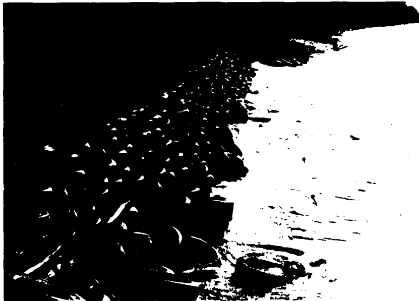
Figure 40 Stacked Used Tire Bulkhead
