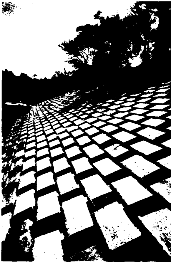
Figure 53 Terrafix Block Revetment
