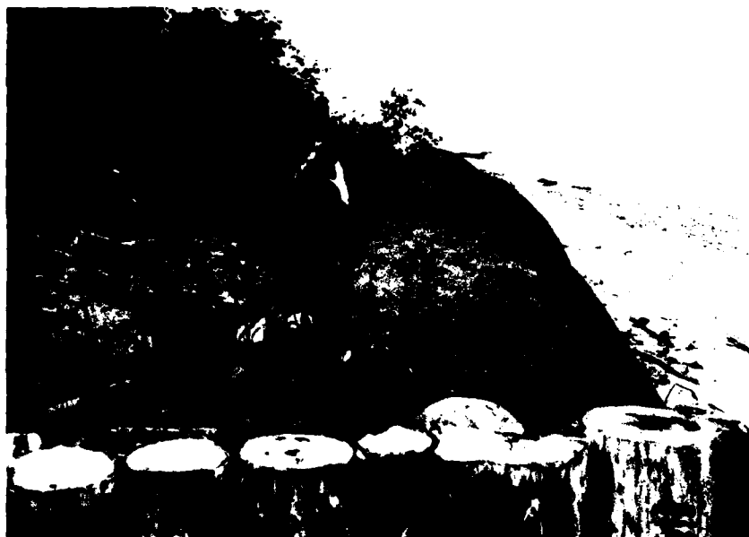
Figure 39 Longard Tube Bulkhead
