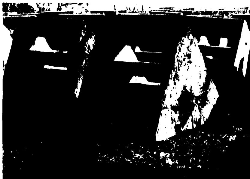
Figure 69 Surgebreaker Modules
