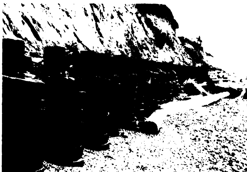
Figure 37 Used Rubber Tire and Post Bulkhead
