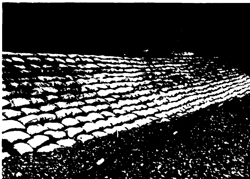
Figure 54 Stacked Bag Revetment
