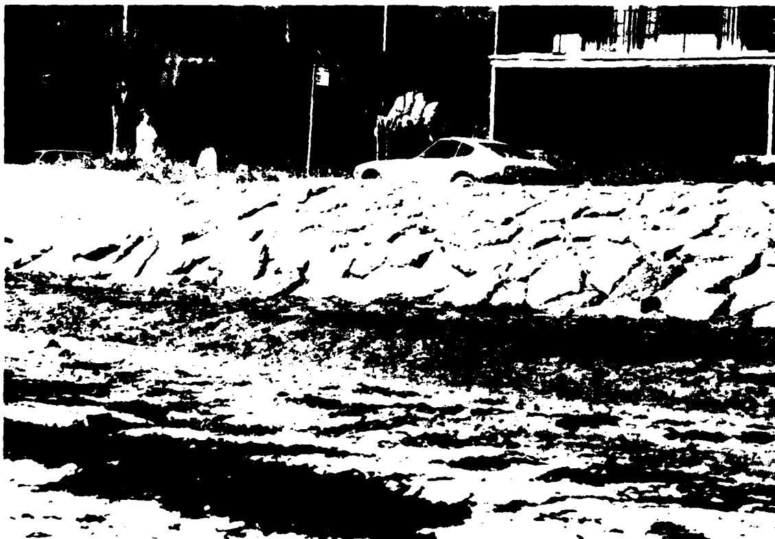
Figure 45 Concrete Rubble Revetment
