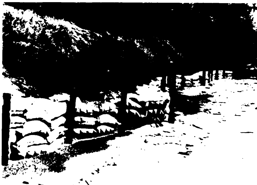
Figure 35 Hogwire Fencing and Stacked Bag Bulkhead
