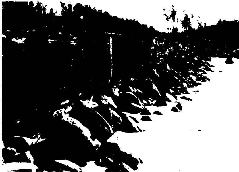
Figure 38 Railroad Ties and Steel H-Pile Bulkhead
