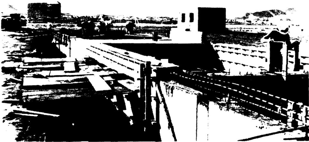
Fig. 5-9. Prestressed Precast Concrete Planks in Areas No. 2 and No. 3.
