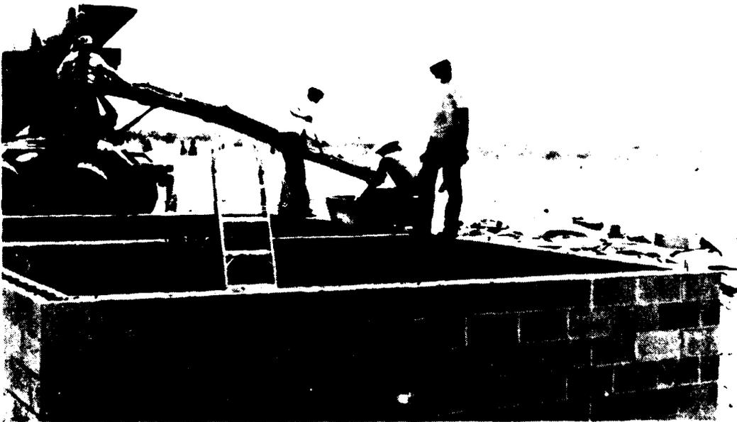
Fig. 4-6. Grouting of Concrete Block Wall.
