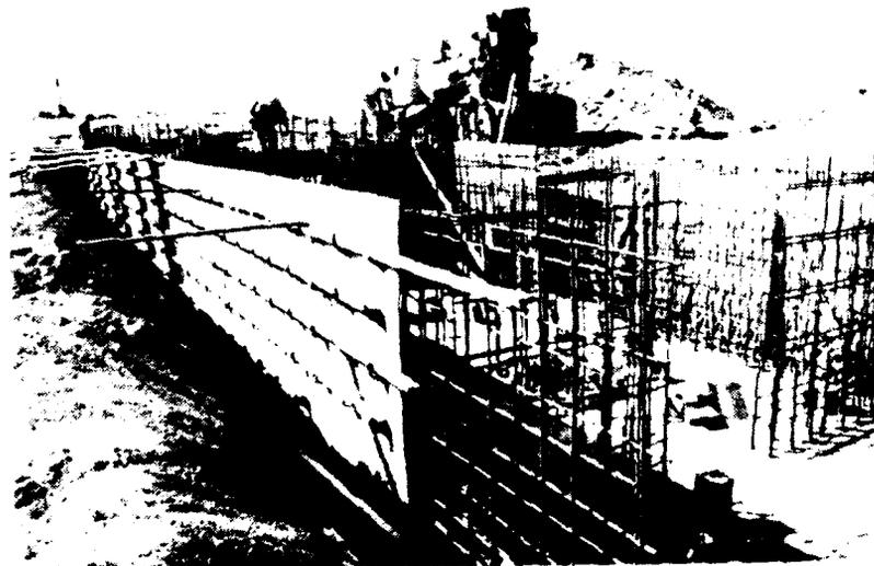
Fig. 5-3. Reinforcing Steel and Forms for Walls.
