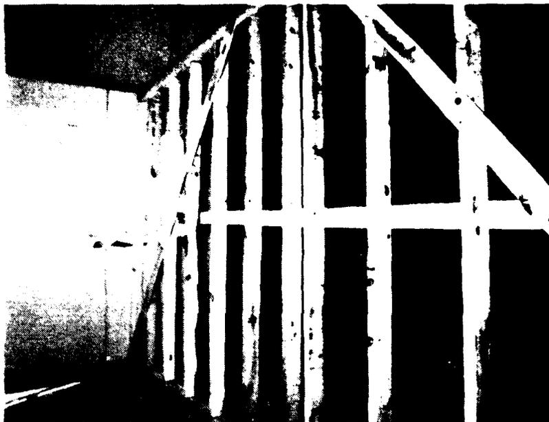
Fig. 2-8. Stud Wall Shoring In Place.
