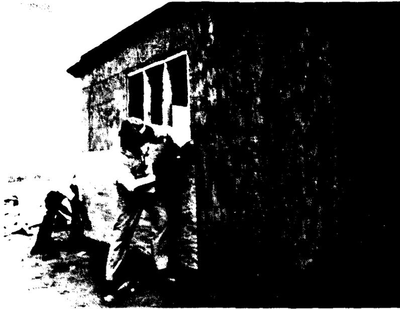
Fig. 2-10. Additional Layer of Exterior Plywood Being Installed.
