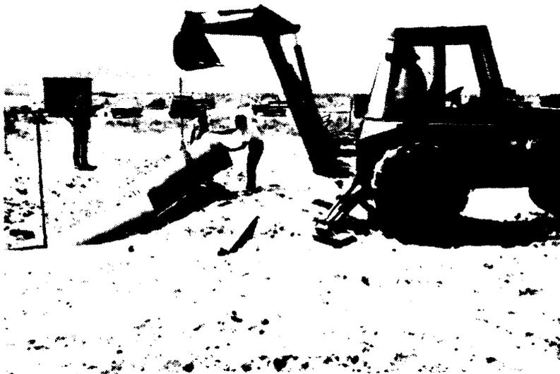
Fig. 6-2. Placement of Concrete Pipe Sections for Access Way.
