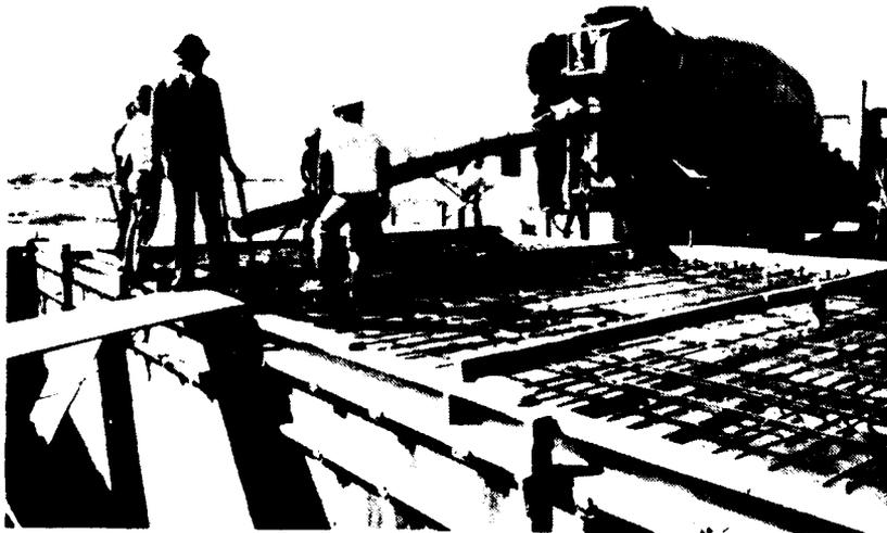
Fig. 5-8. Concrete Deck in Area No. 1 Being Placed.
