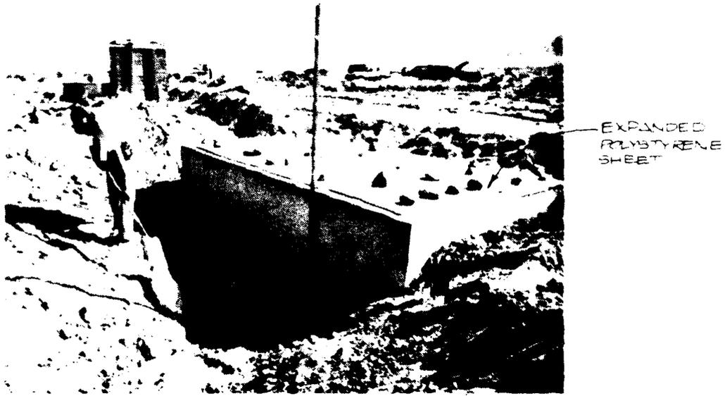
Fig. 6-4. Roof of Vault at 40 psi Environment.
