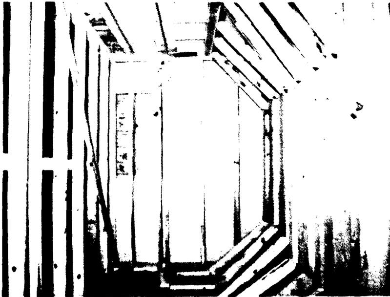
Fig. 2-11. Interior of Building With Shoring and Closures.
