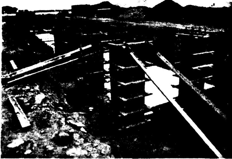
Fig. 5-7. Forms for Columns and Pilasters in Area No. 4.
