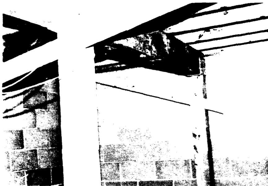
Fig. 4-8. Posts and Beam in Position.
