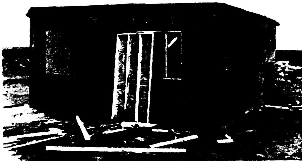
Fig. 2-9 Door and Window Closures Partially In Place.
