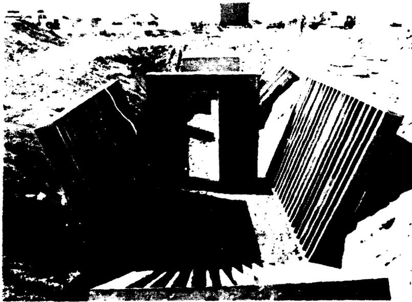
Fig. 8-7. First Stage of Assembly of Shelter.
