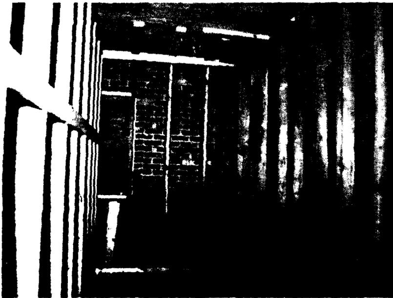
Fig. 3-9. Stud Wall Shoring and Wall Bracing, Pretest.
