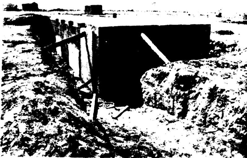
Fig. 5-12. Completed Structure Partially Backfilled.
