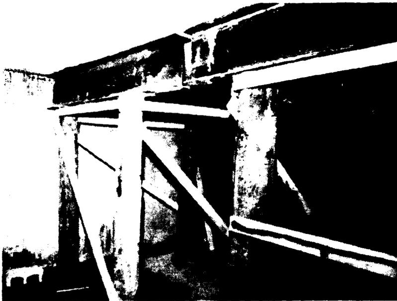
Fig. 5-18. Post and Beam Shores in Area No. 2.
