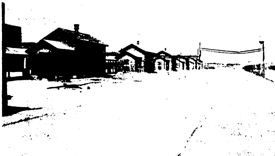
Figure 15b. Inactive operations buildings, "400 Area".
