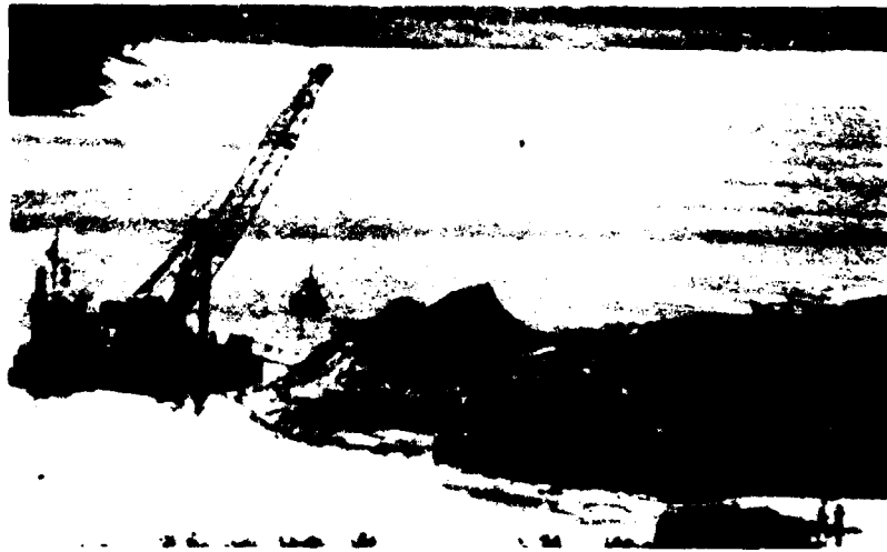
Figure 6. The Clamshell Dredge Derrickbarge 771 Redredges the Spoil Dropped by the Barges and Casts it on to the Spoil Bank. Note the Figures in the Right Foreground (Colingsworth)
